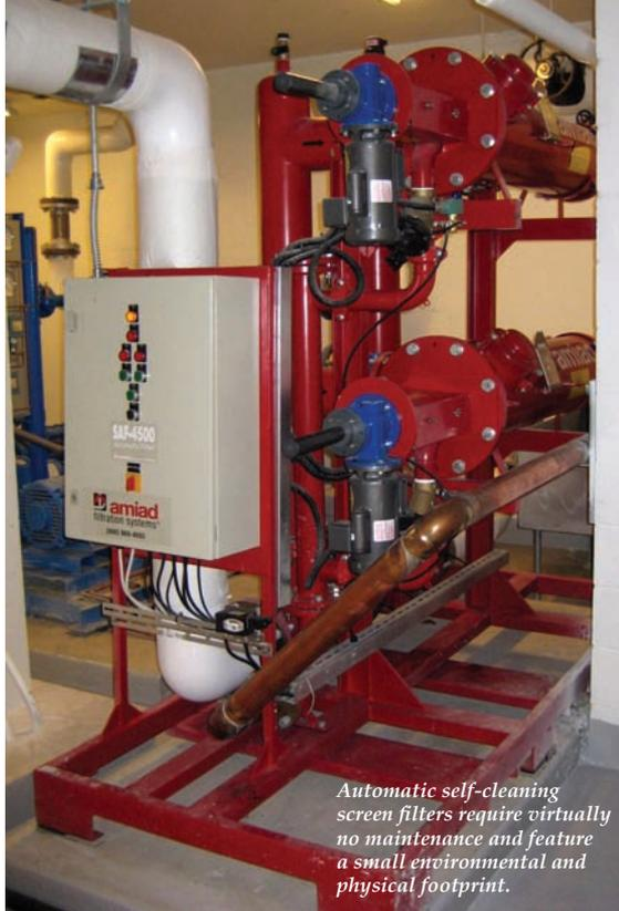
*Automatic self-cleaning screen filters require virtually no maintenance and feature a small environmental and physical footprint.*
