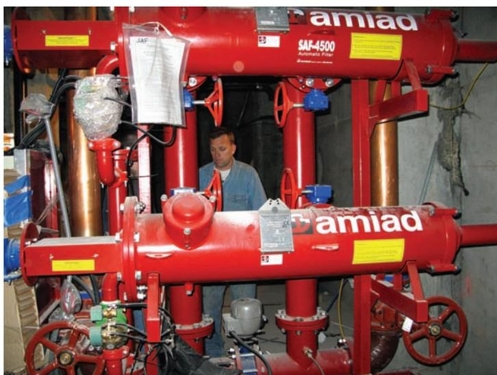
Screen filters operating at the 10-micron level at the domestic water supply's point of entry can triple the life of 0.2-micron point-of-use filters in individual apartments.
